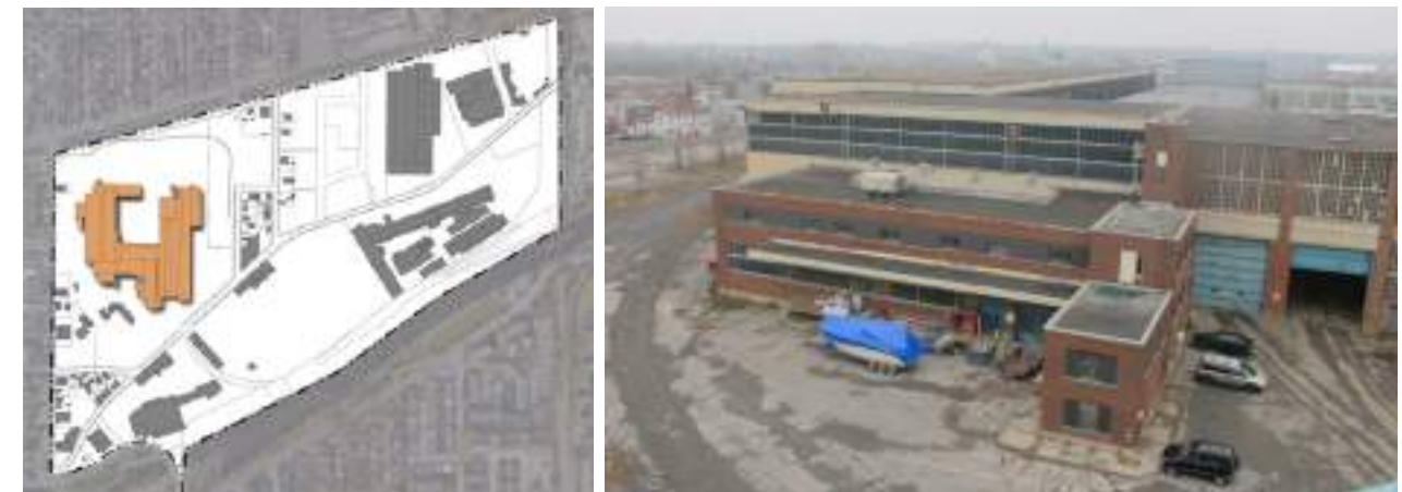
Figure 4: Emplacement et photo de Dominion Bridge (Culture et communications Québec, s.d.)
